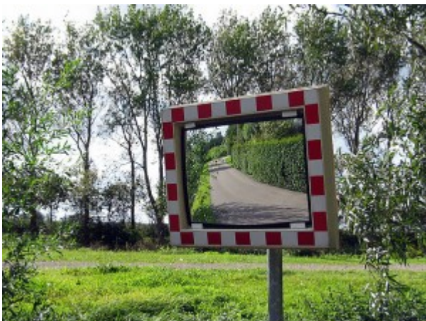
Image : Convex mirror for an overview of road traffic. By Gerard Hogervorst, License: CC BY-SA 3.0
